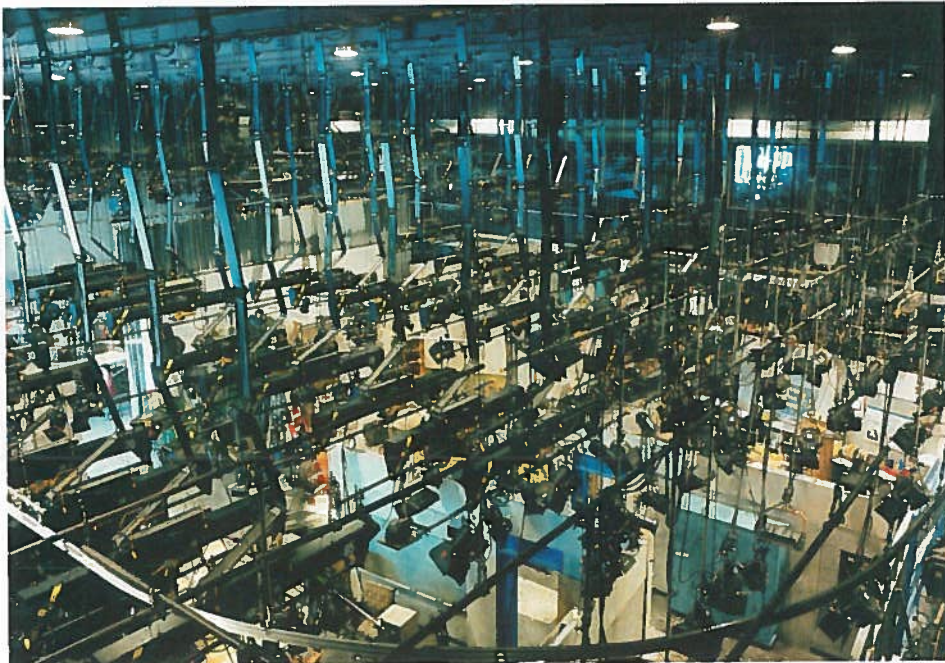
1990: 200 self-climbing hoists were supplied to studios 18 and 19 at Universal Studios, Orlando.
